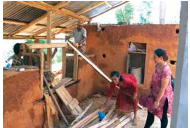
Khadka Kumari, in rebuilding her house, Sarki Gaun, Sindhupalchowk
